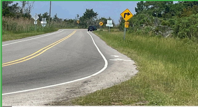
28 Existing Bike Lane on Fort Fisher Blvd
